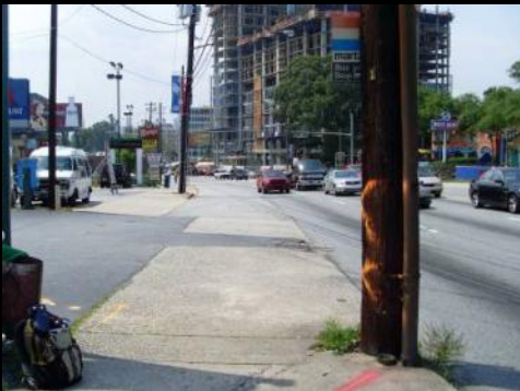
Along parts of the segment, there are times that the sidewalk height is even with the roadway height, creating essentially a continuous curb cut, with no separation between pedestrians and automobiles.
