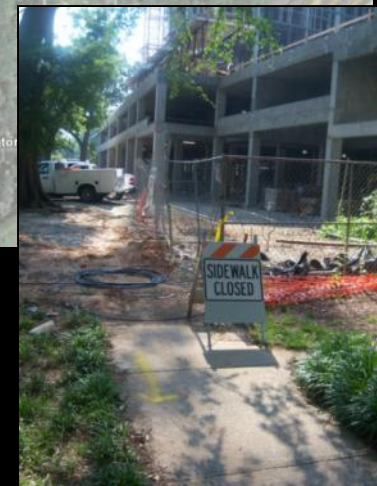
Closed sidewalk due to construction on The Brookwood condominiums.
